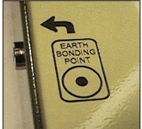
The earth bonding point can be used to plug in an anti-static wristband conforming to EN100 015-1.
